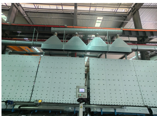
1#密封胶废气集气罩
